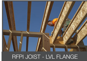
RFPI JOIST - LVL FLANGE
